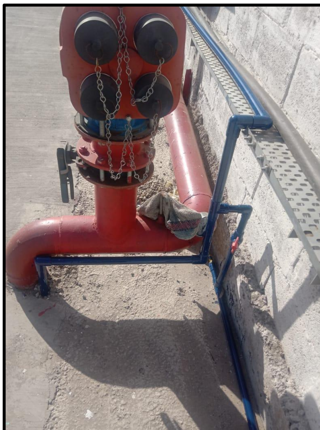
Color Coding Provided for Pipelines
